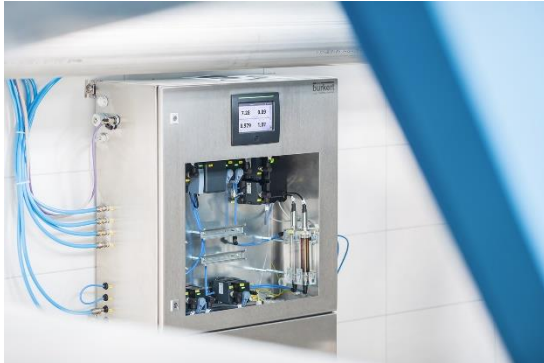
Image 1: Type 8905 online analysis system offers automated water quality monitoring for a wide range of applications.
