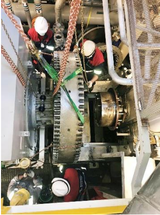
Image 1: Burckhardt Compression experts working on the compressor skid in the confines of the compressor machinery room (CMR).
