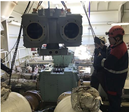
Image 2: Re-assembly of compressor.
