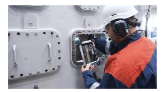
**Image 3:** Including within the package is an ATEX-certified tablet and headset that enables the technician on-site to communicate and receive instructions via a secure network connection.
