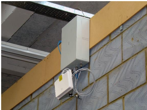
Image 1 – Enclosures IP rating to protect the Wi-Fi access point inside the enclosure from water damage.
