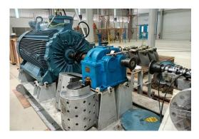
**Image 3:** The old diesel drives and steam turbines were replaced with new electric motors and gearboxes to deliver the desired speed increase.
